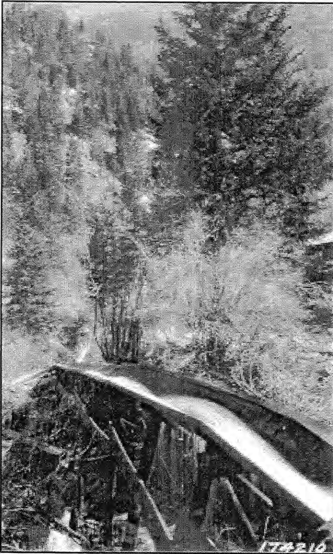
Intake for adding water to log flume father down the canyon. Photograph courtesy the U.S. Forest Service.
