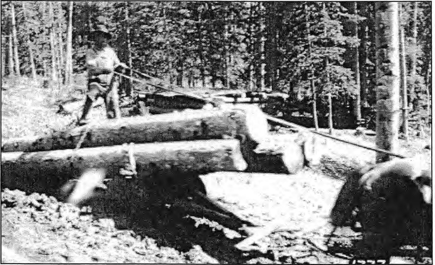
Skidding logs to the railroad using a "bummer." Note the crude wheels under the front of the logs. Photograph courtesy of the U.S. Forest Service.
